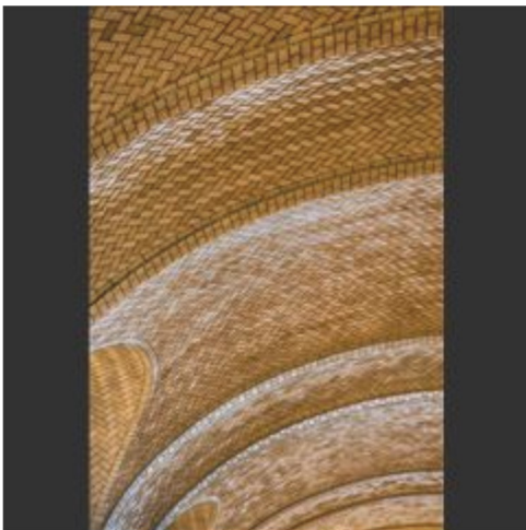
Lines Proj Guastavino Catalan Vault Ira Nemeroff
