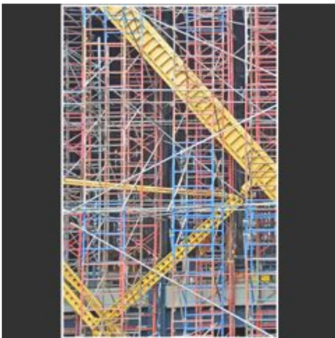
Lines Proj Construction Pattern David Patterson
