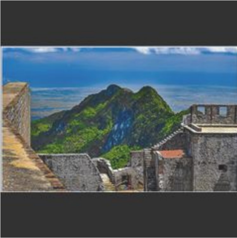
Advanced Proj Citadel Vantage Point - Haiti James Bashant
