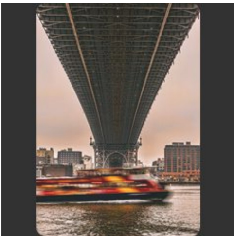
LCC-5 Class-A Proj Under The Bridge Howard Hoffman TA
