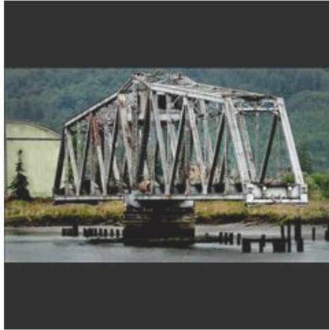
Advanced Proj Bridge to Nowhere Jean Fingerhut
