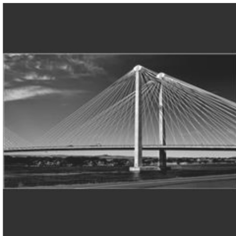
Advanced Proj-Mono Cable Bridge Jean Fingerhut
